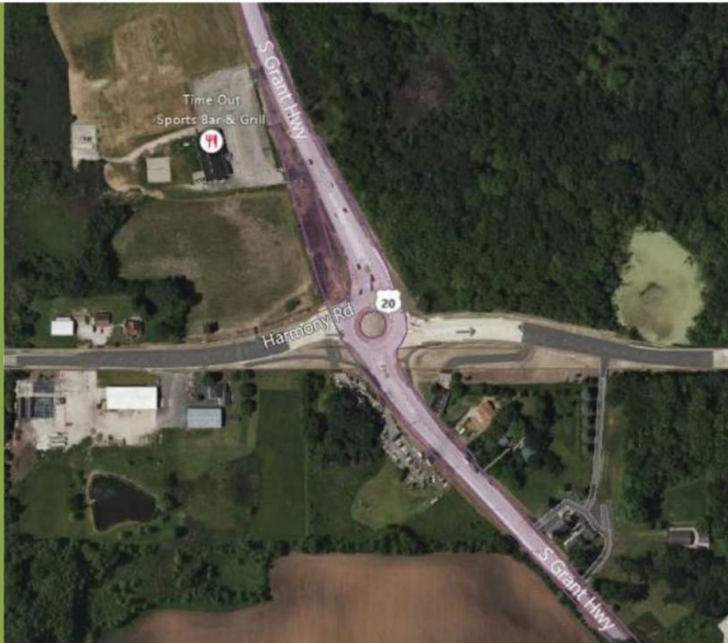
US 20 AND HARMONY ROAD Year of construction: 2018-2019
